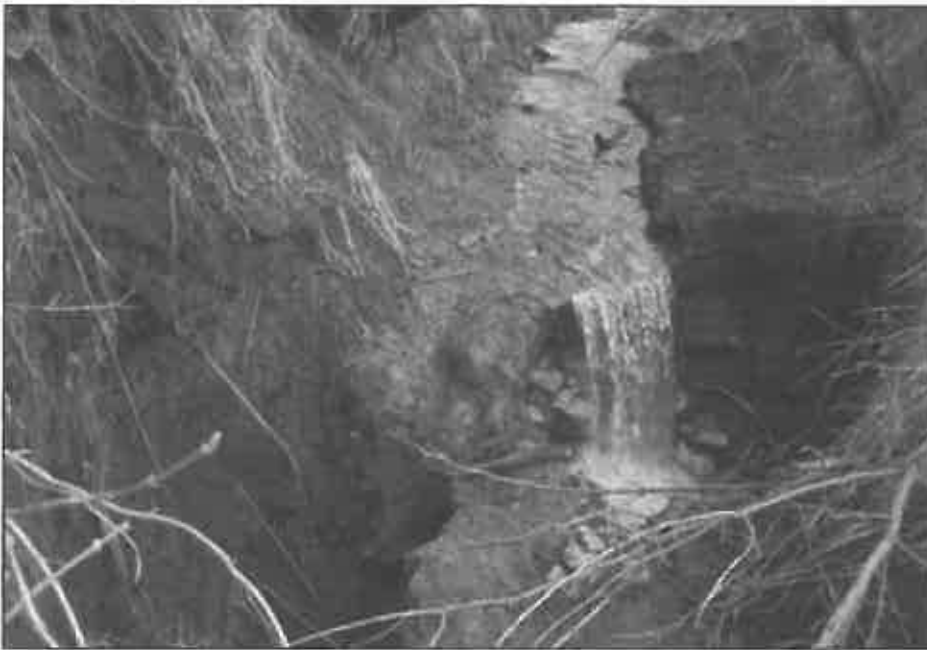
Figure 2-2. In-stream sinkhole in Silver Creek.
